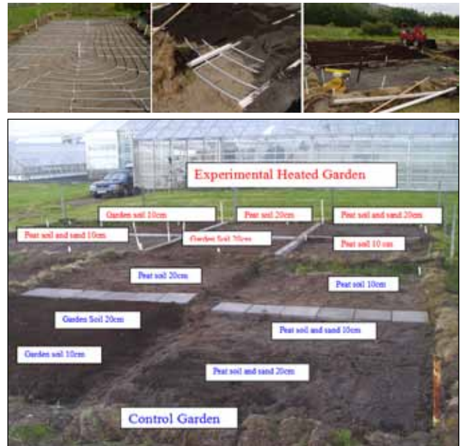
Figure 2: Hveragerdi spiral piping layout (top left), sand over layer construction detail (top center), soil top layer and gravel compaction construction detail (top right), soil depths, types and location (Bottom)
